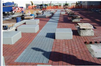
Substitute Tufchem™ Grout, Acrocast™ Polymer Concrete, or Pennchem™ Novolac Grout for Portland cement concrete pads, piers, and footings in corrosive service.
