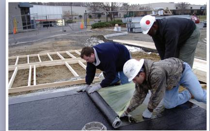
To waterproof elevated slabs, select from a versatile range of asphaltic membranes: hot melt Penncoat™ 101 Membrane, cold-applied Tufchem™II Membrane, or adhesively bonded Penncoat™ 600 Membrane sheet.
