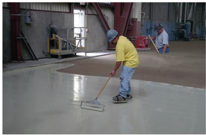
Pennrowel™ Systems trowellable, slurry-broadcast, and laminate polymer linings provide durable corrosion protection for floors and other concrete structures.
